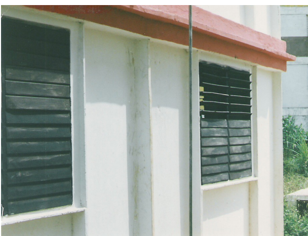
Three-storey building, more than 20 years old
