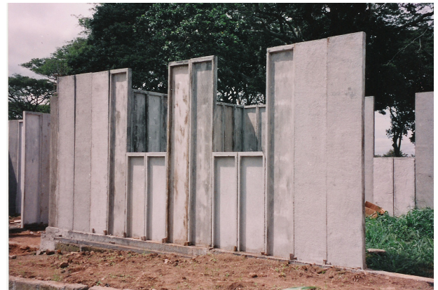
placing the elements on U-shaped beams
